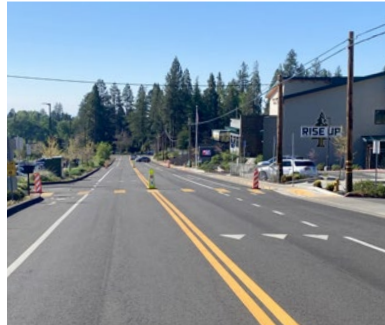
“Rise Up:” Knife River helped rebuild critical roadways in Paradise, California, after the Camp Fire.
